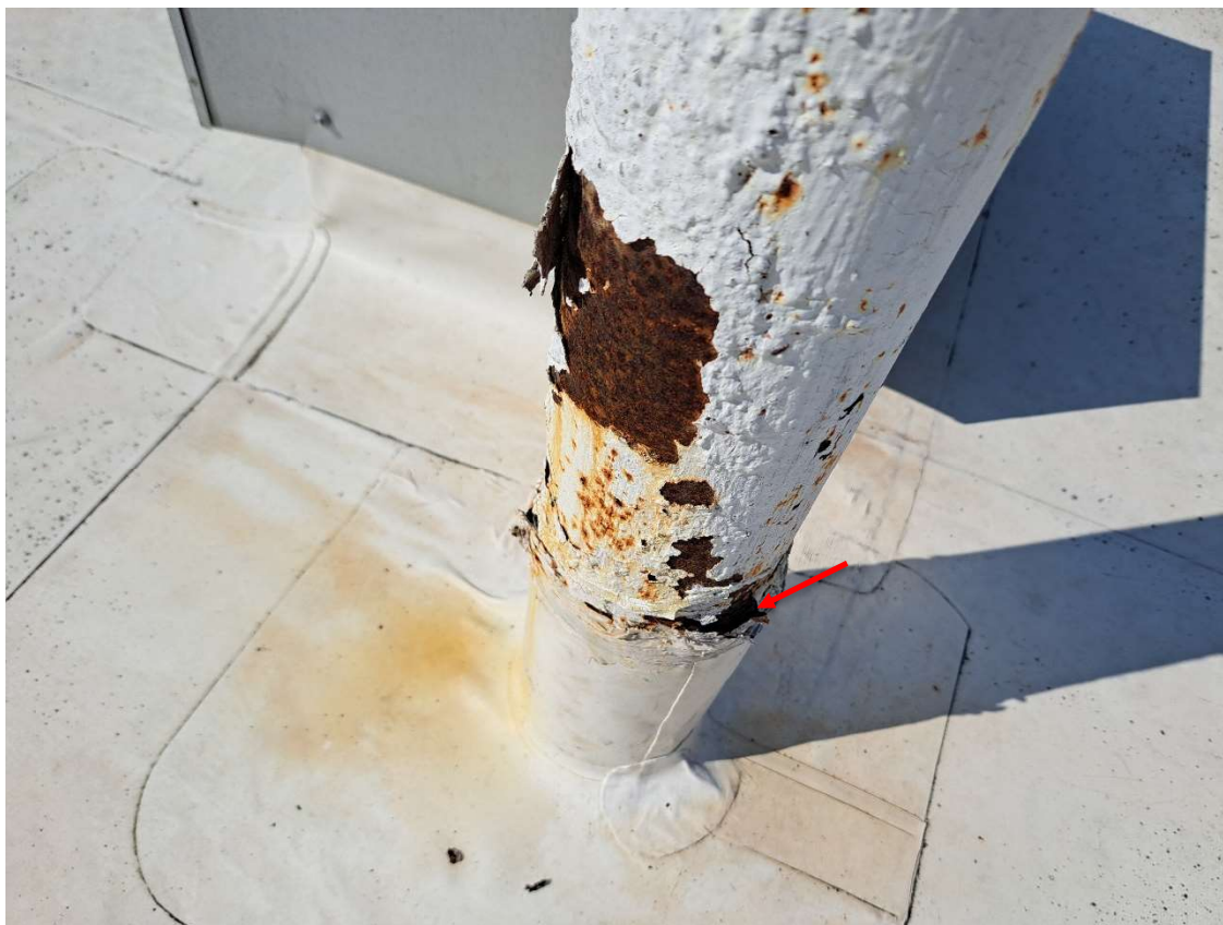
Photo 06 Ref: 2.1.2.1 – Damaged Upper Flashing of the Fire Hydrant Pipe on the Roof
