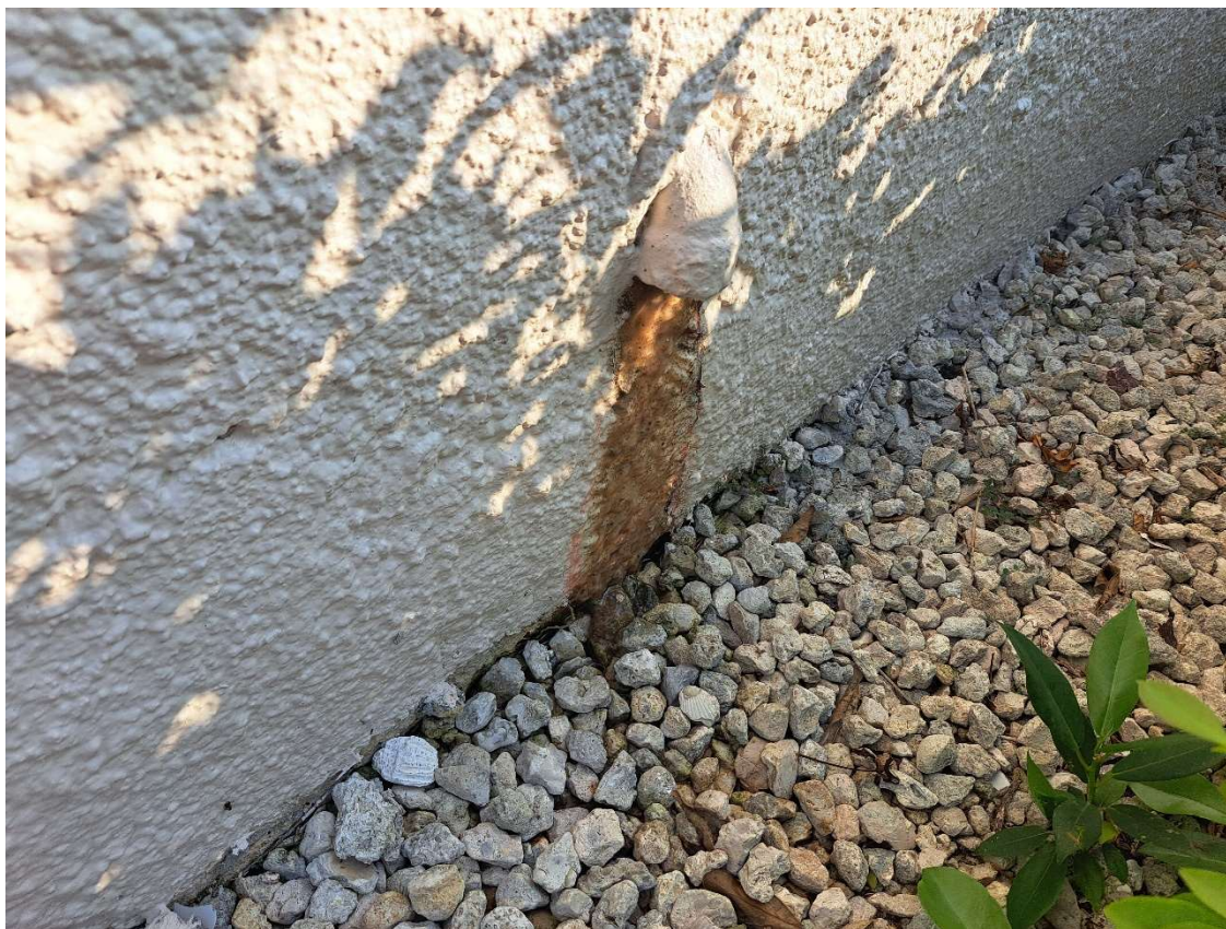
Photo 05 Ref: 2.1.1.1 – Downspouts Draining Next To Foundation
