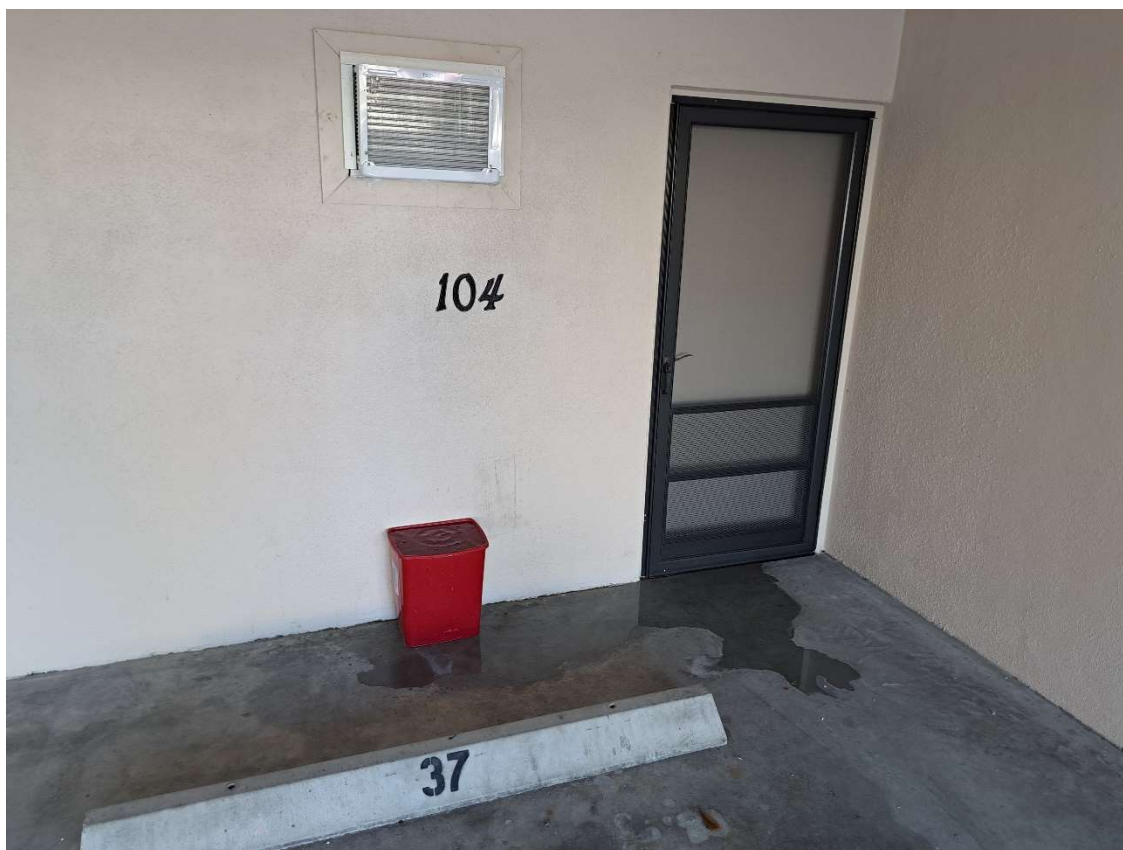
Photo 01 Ref: 2.1.1.1 – Air Conditioner Condensate Draining Directly Onto Floor
